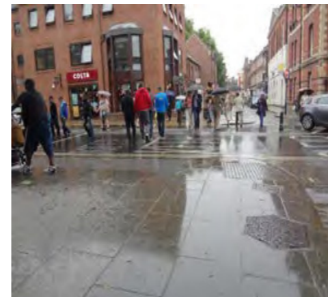
A very good example of a crossing with English Pennine sandstone blister paving on Museum Street
