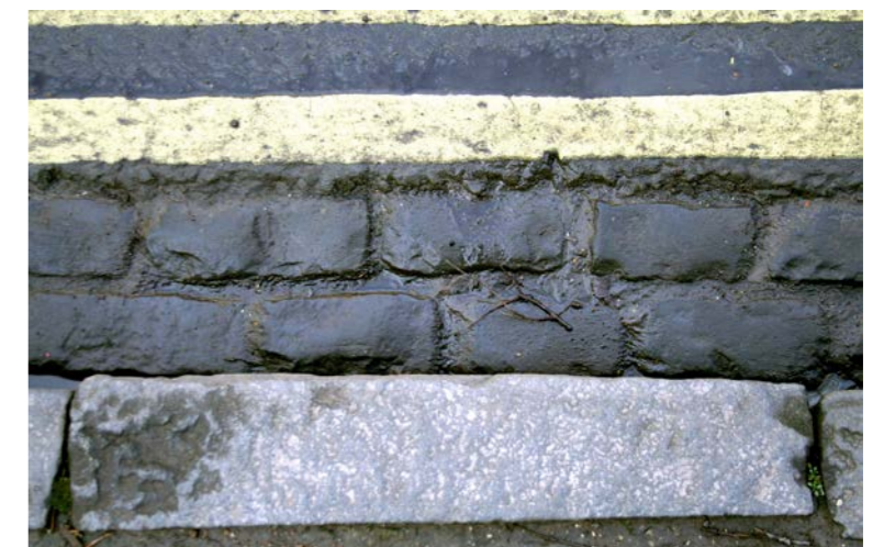
Brick drainage channel and granite kerb with neatly laid asphalt.
