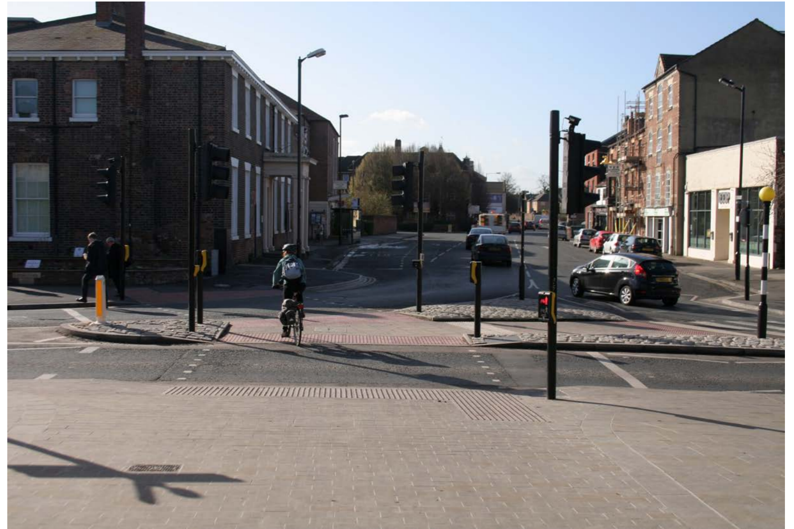
The recently (2013) re-designed crossing at the junction of Paragon Street and Fawset Street demonstrating significant improvement in cycle and pedestrian experience on the inner ring road.
