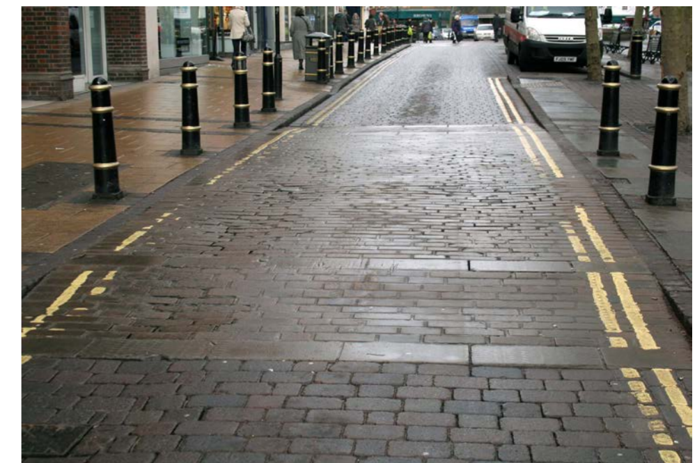
A well constructed raised table on Parliament Street consisting of English Pennine sandstone setts with pre-cast brick paviours on either side, providing level access across the carriageway.
