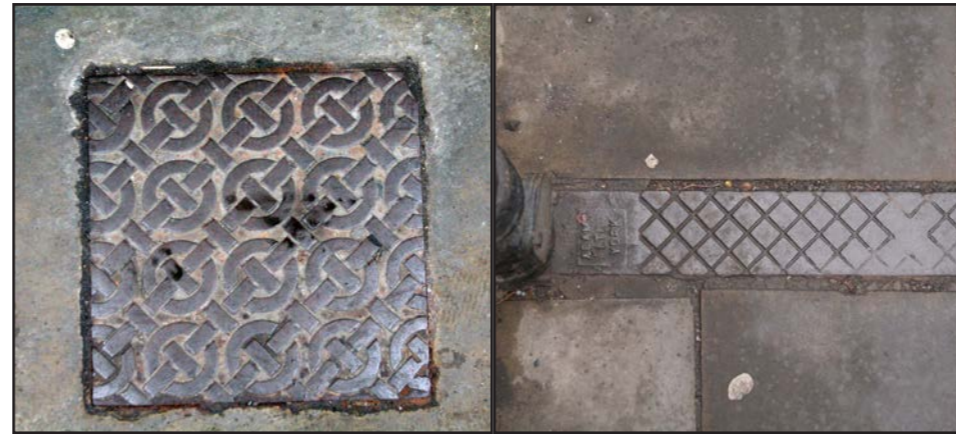
Two types of cast iron feature - on the left, an inspection cover by Dove and Sons, and on the right a cross footway rainwater channel by William Kirk.
