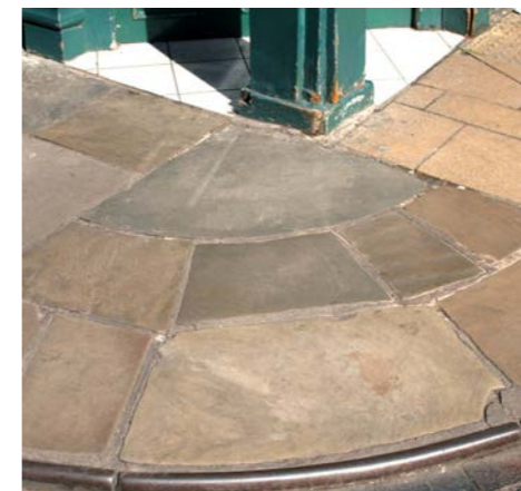
Well thought out approach to laying riven flags at a corner - note the original cast iron kerb, used to protect the pavement edge
