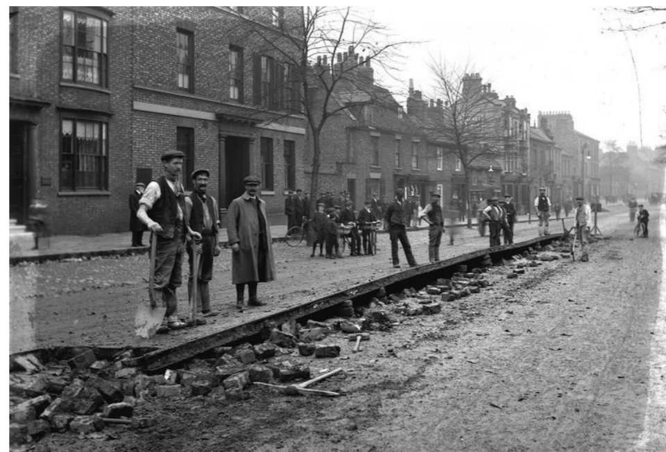
This photograph records a pause in electric tram track laying on Blossom Street in 1910, clearly showing stone setts, later replaced. (City of York Archives)
