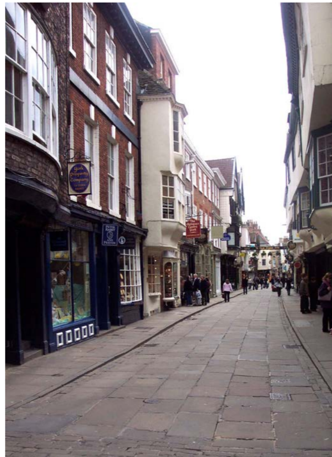
Stone flags on Stonegate carriageway.
