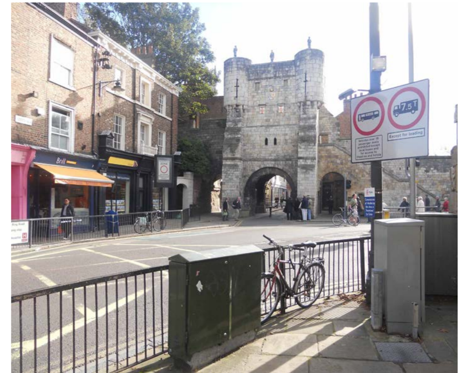
Railings at Bootham Bar - poor quality and combining with too many utility boxes significantly impacting on the setting of this important gateway into the city
