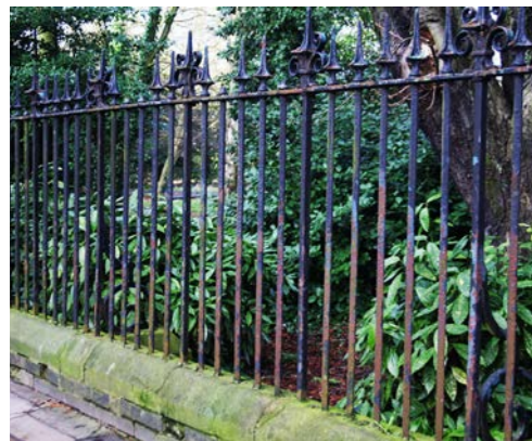
Listed railings at Bootham Hospital
