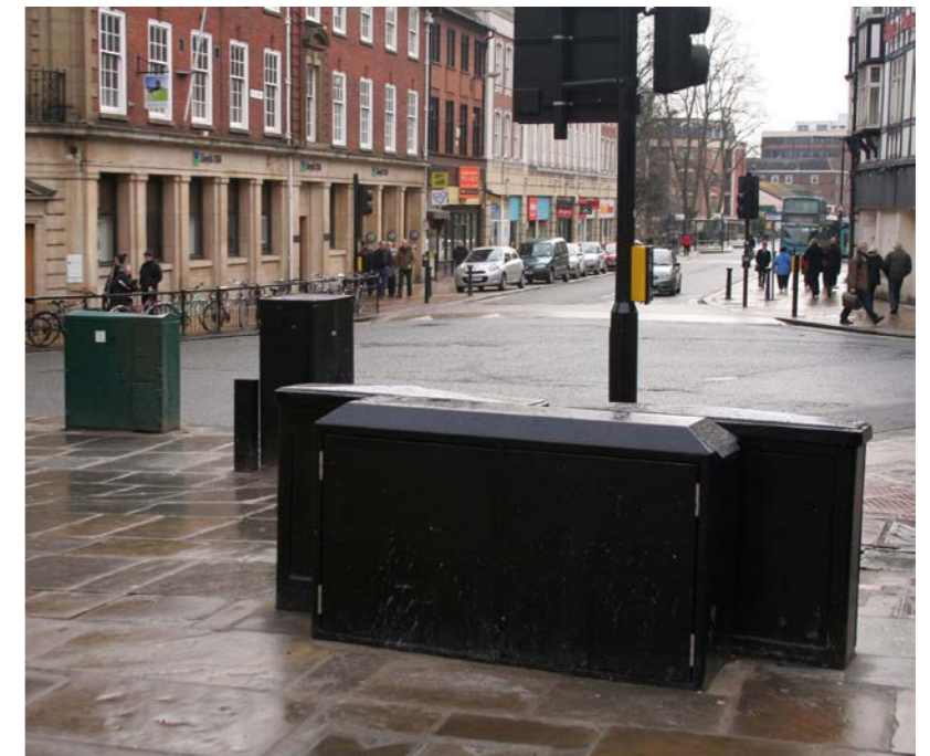
An unfortunate collection of cabinets in black and green at the junction of Parliament Street, Pavement and Piccadilly. Opportunities to rationalise this situation should be taken with utility companies and the Council's Network Management function.
