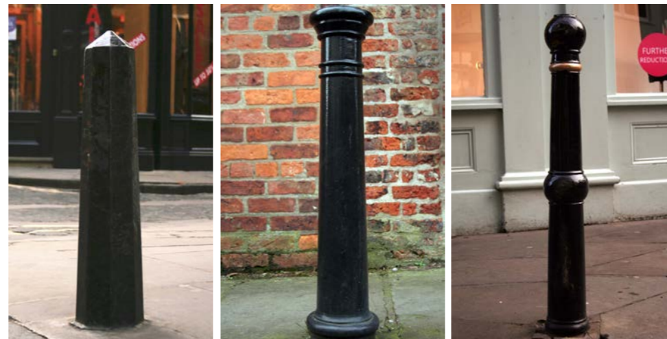
Selection of bollards in use in the city centre with the so-called York bollard on the left
