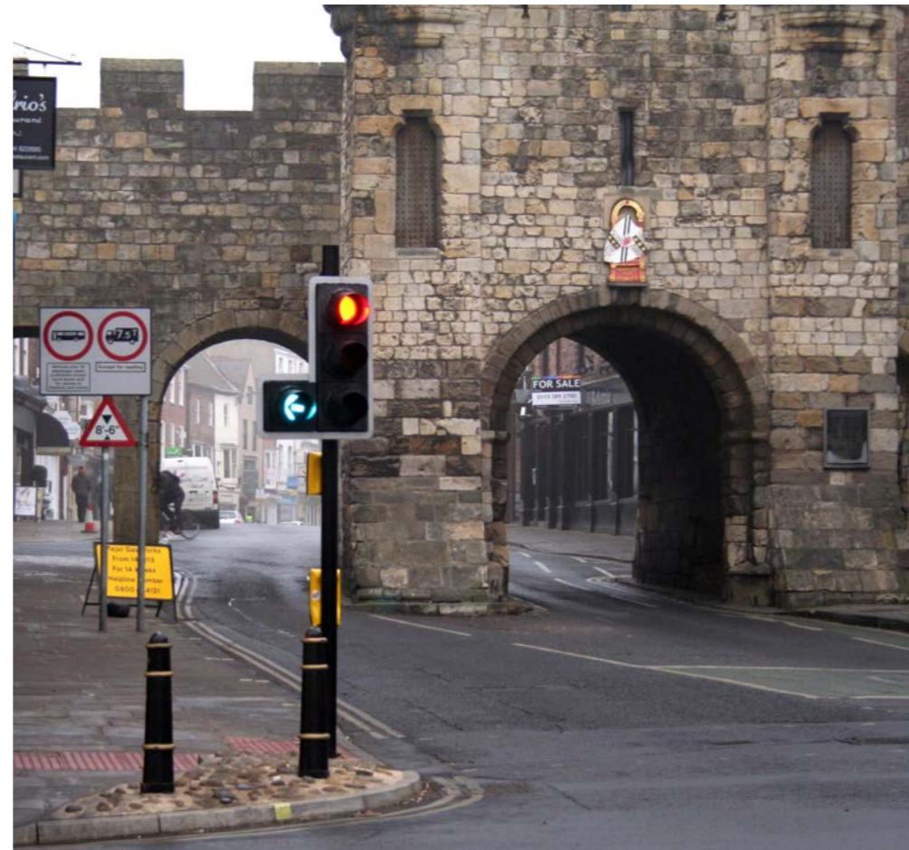
Secondary traffic lights adversely affecting the setting of Micklegate Bar
