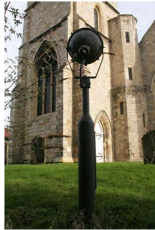
An elderly floodlight with a high pressure sodium luminaire aimed at the tower of St Deny's Church, Walmgate
