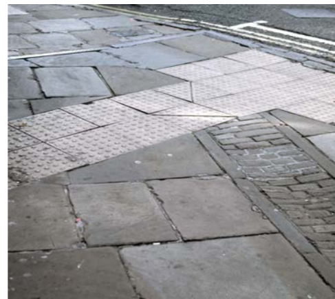
Poor use of tactile paving in King's Square where it is not really needed
