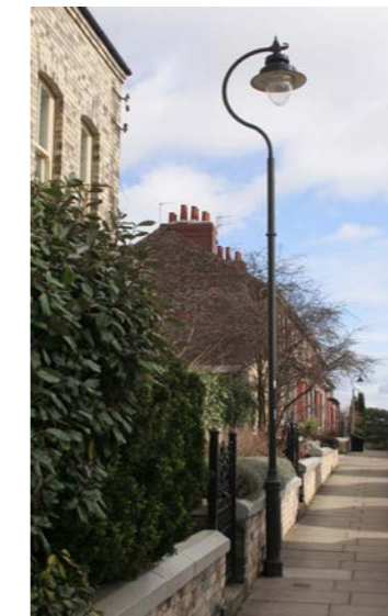
Traditional decorative cast iron column with a swan neck and replica globe lantern in Bishophill
