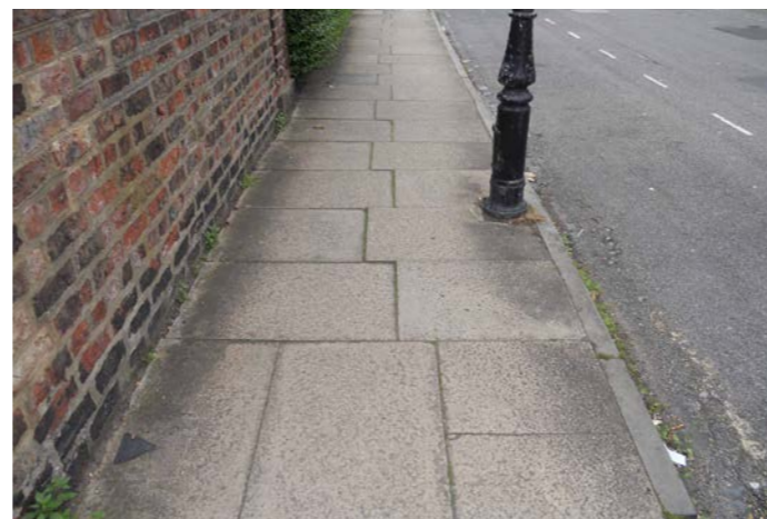
Although replacing traditional riven Sandstone flags, these staggered 1950s concrete paving slabs in Bishophill are more preferable to contemporary smaller pre-cast paving.
