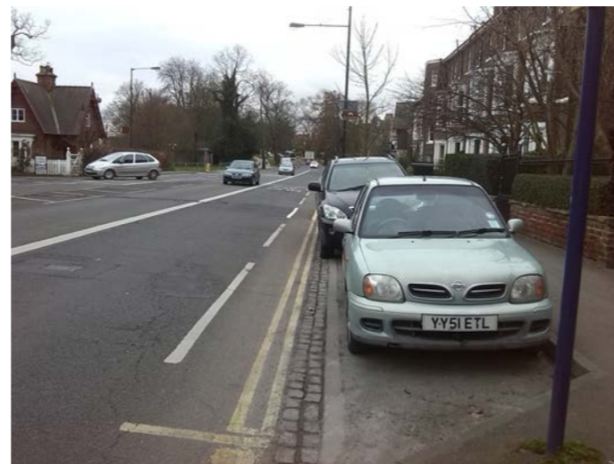
Vehicle parked within a roadside bay with wing mirror and off-side wheels projecting onto a cycle lane - The Mount (cycle lane is 1.1m wide).
