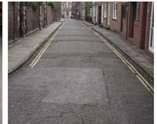
Asphalt carriageway surface in Aldwark with mixed aggregate inclusions providing an attractive variant to more ubiquitous plain asphalt surfacing
