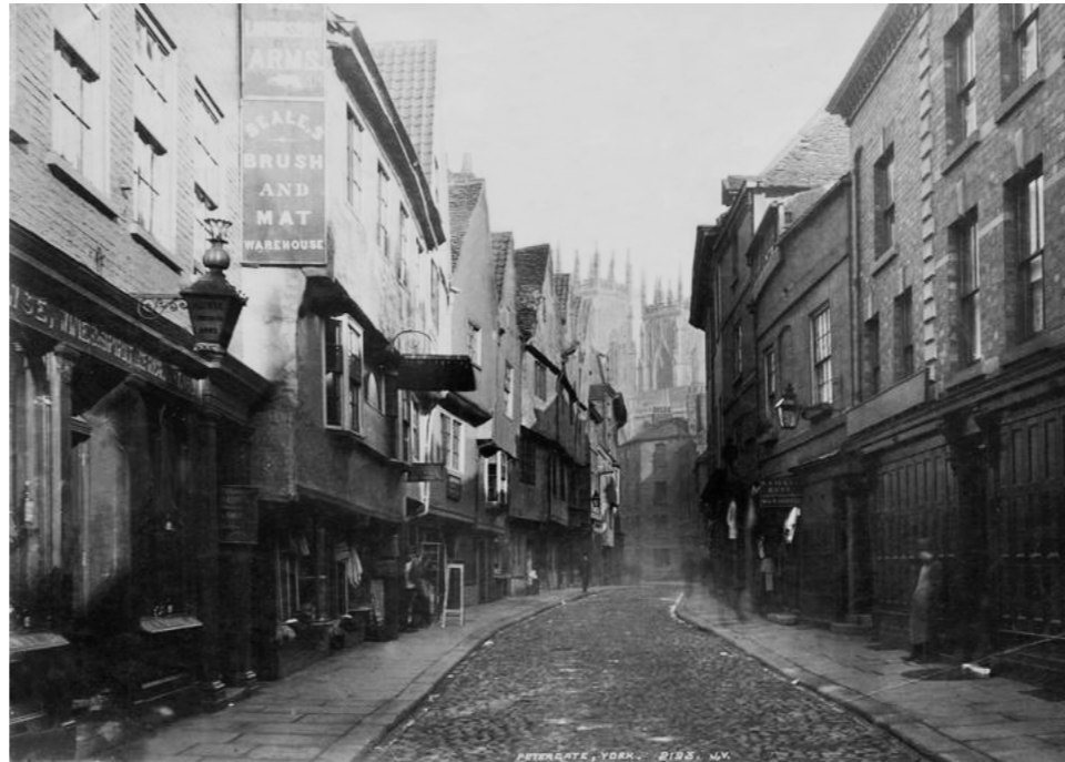
This 1880s photograph of Low Petergate shows the relationship between flagstone pavements, a good wide stone kerb and the carriageway with stone setts - all locally sourced English Pennine sandstone. (City of York Archives)
